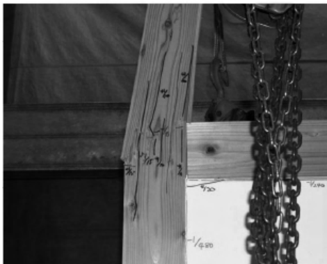
(c) 窓台部中柱曲げ破壊
