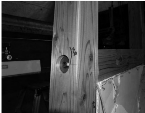
(c) 窓台部中柱曲げ破壊
