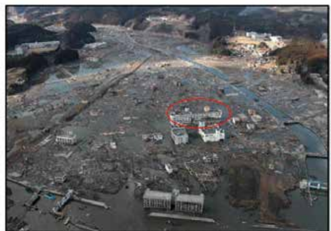
Shizugawa Hospital, Minamisanrikucho, Miyagi (2011/3/12 Sankei Newspapers)
